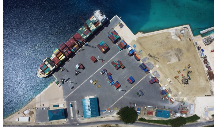
Newly Built Lapetasi Wharf 2018
